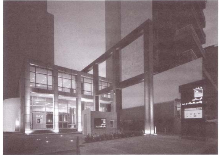
View of the building from the main street
